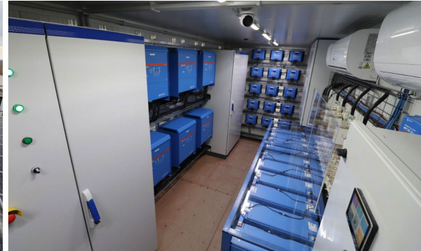
Containerized Power conversion 90kVA DC+40kVA AC and Storage 100kWh
